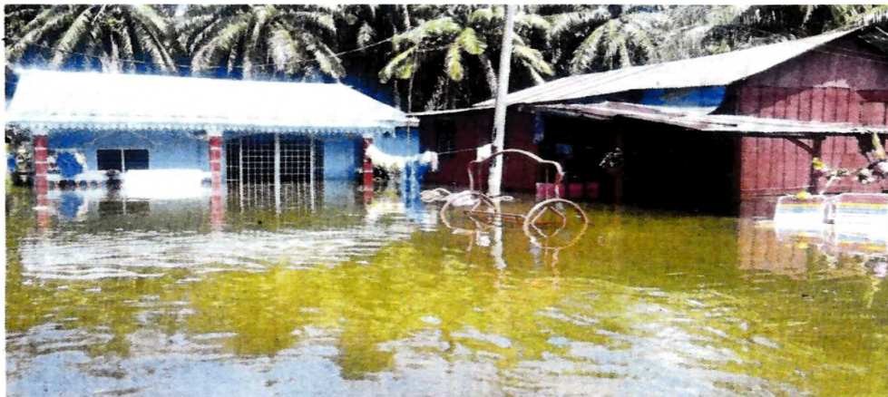
Houses inundated by floodwaters in Changkat Jong , Teluk Intan, Perak. Pic courtesy of the Fire and Rescue Department
